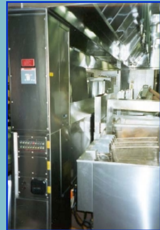
Food-preparation equipment drawing large loads is located along the Energy Wall for easy access in case of tripped circuit breakers
